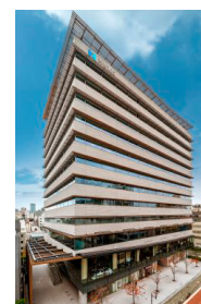
Hulic Asakusabashi Building
