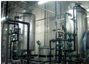
State of installation of subway seep water filtration system (Ochanomizu Sola City)
