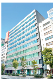
Hulic Toranomom Building
