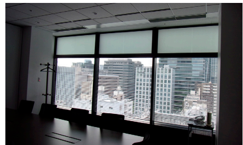
Natural lighting film (Hulic Toranomon Building)
