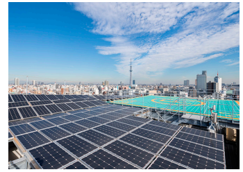
Hulic Asakusabashi Building
