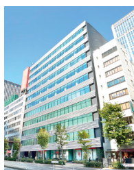
Hulic Toranomom Building
