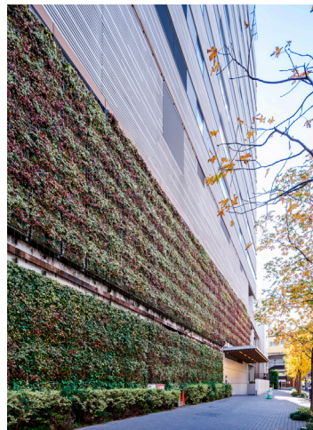
Hulic Asakusabashi Building
