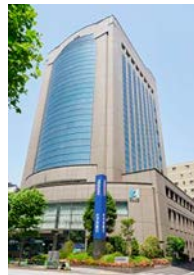
Hulic Kobunacho Building
