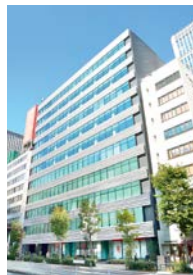
Hulic Toranomom Building
