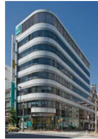
Hulic Higashi Ueno 1 Chome Building
