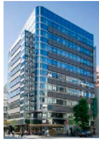
Hulic Kakigaracho Building
