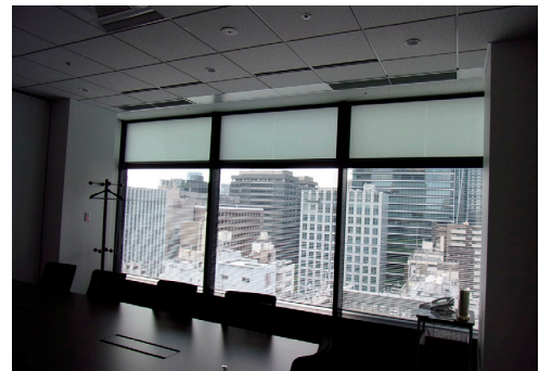
Natural lighting film (Hulic Toranomon Building)
