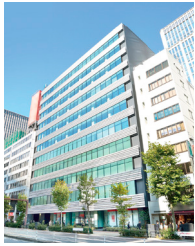
Hulic Toranomom Building
