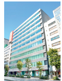
Hulic Toranomon Building
