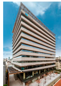
Hulic Asakusabashi Building
