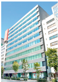
Hulic Toranomom Building
