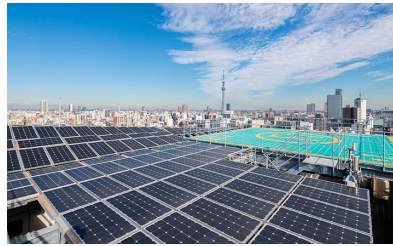
Hulic Asakusabashi Building
