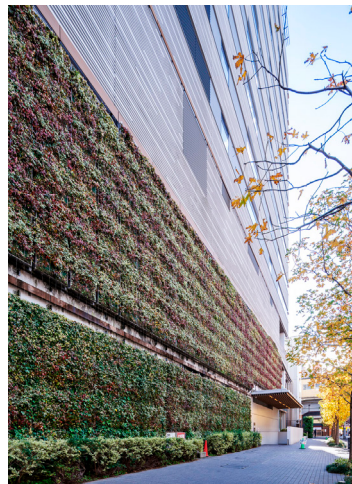
Hulic Asakusabashi Building
