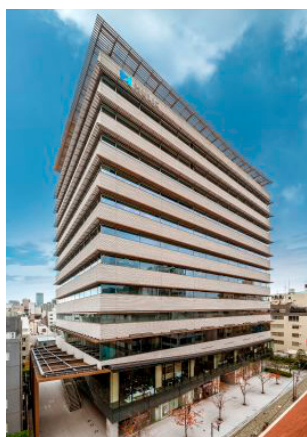
Hulic Asakusabashi Building
