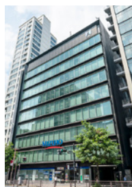
Hulic Kojimachi Building
