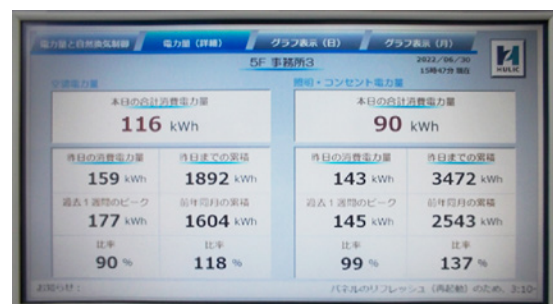
Energy management tool (Hulic Asakusabashi Building)
