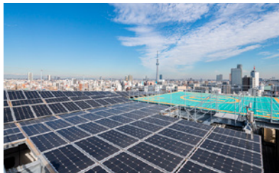
Hulic Asakusabashi Building
