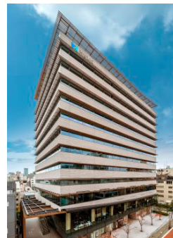
Hulic Asakusabashi Building (acquired in December 2019)
