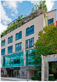
Hulic Jingumae Building
