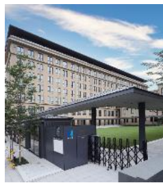
Rissei Garden Hulic Kyoto (THE GATE HOTEL Kyoto Takasegawa by HULIC)
