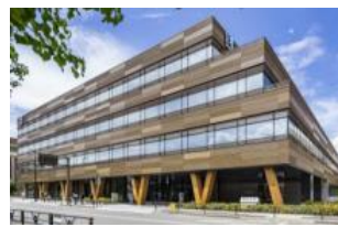
Hulic Shogi-Kaikan Sendagaya Building
