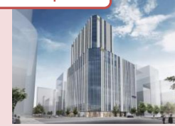
HULIC SQUARE SAPPORO (Phase II) (Sapporo Building Reconstruction Project) (2025)
