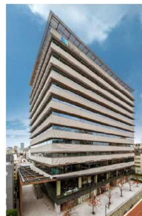
Hulic Asakusabashi Building
