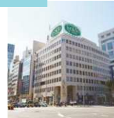
Hulic Aoyama Building
