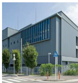
NW-08 Network Center
