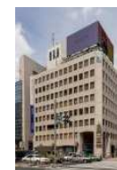
21 HULIC Aoyama Building
