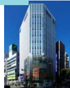
Hulic Shinjuku Building
