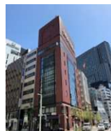
3 Ginza Tenkuni Building
