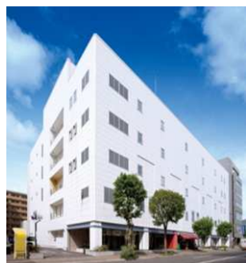
NW-07 Network Center
