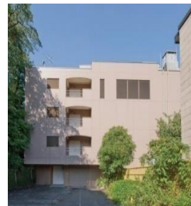
NW-02 Network Center
