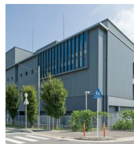
NW-08 Network Center
