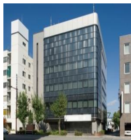
NW-05 Network Center
