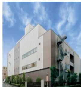
NW-01 Network Center
