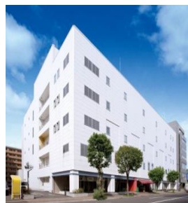
NW-07 Network Center
