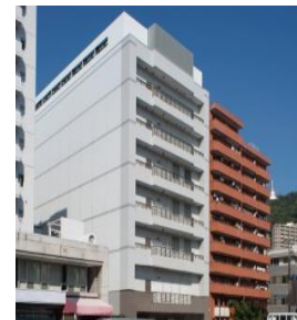
NW-03 Network Center
