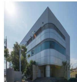
NW-04 Network Center
