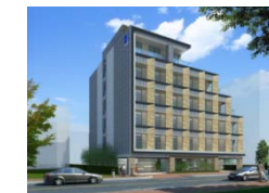
Shibuya Higashi 4 Chome Development Project (Private nursing home)
